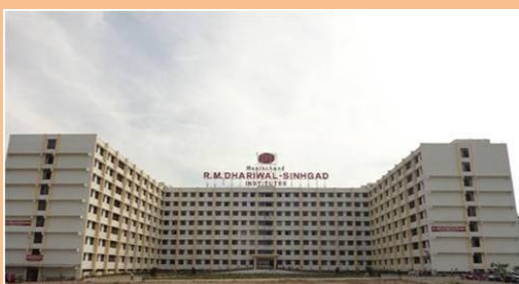
RMD Sinhgad School of Management Studies Campus, Warje, Pune
